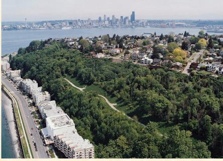
East facing view of Alki Landslide after remediation with 1/4 mile long interceptor drain and horizontal drains. Photo submitted by W.T. Laprade.
