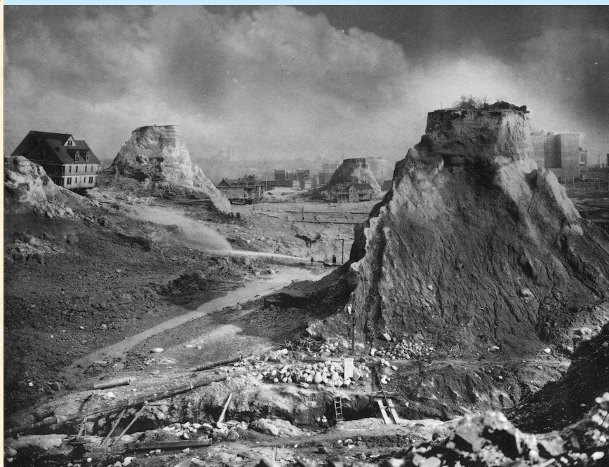
The 4th Denny Regrade, which removed 5.5 million yds 3 of sediment and dumped it in Elliott Bay. Photo by Asahel Curtis, c. 1910.
