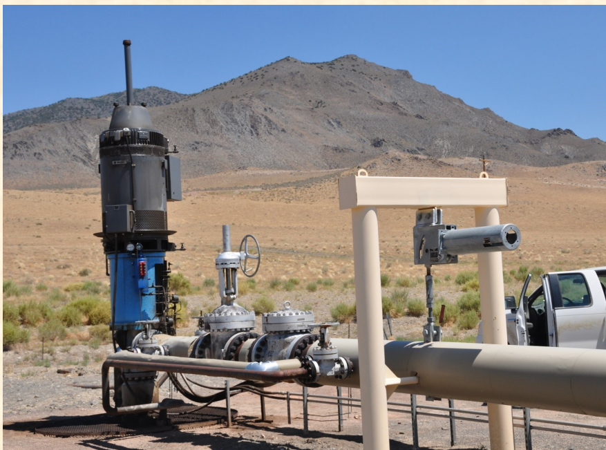
Photo of pipeline and 700 HP, electric motor driving a line-shaft pump set at 1700 ft below ground surface. The pump produces 2000 gpm of 320 F water. It is one of 6 pumps at Blue Mountain Geothermal Field, a 29 MWnet power plant 30 miles west of Winnemucca, NV.
