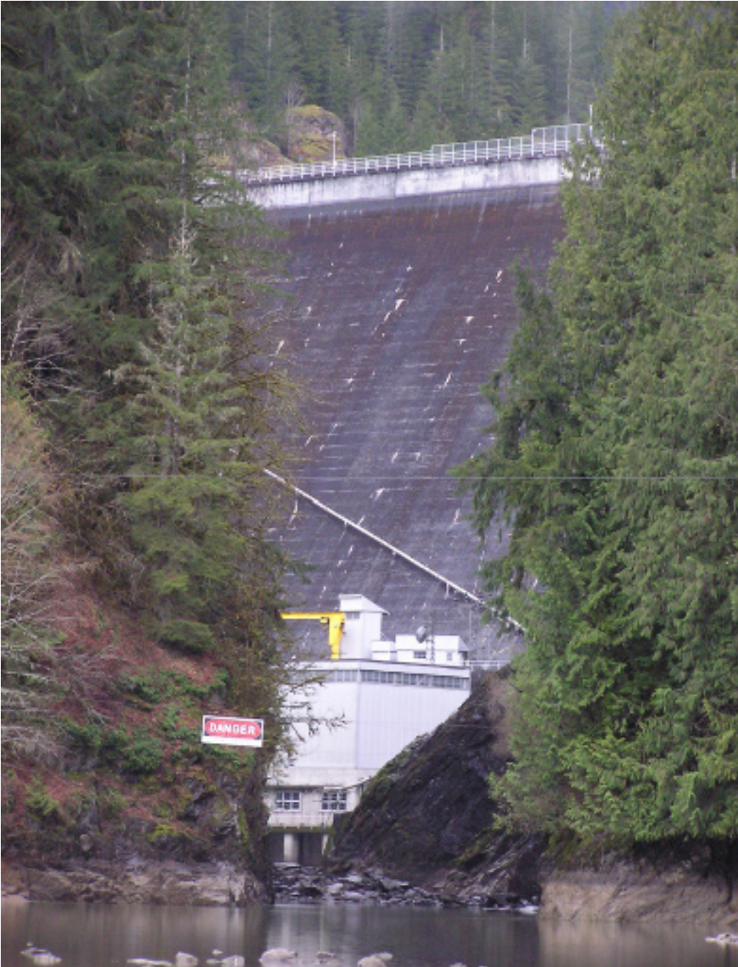
Figure 7. The downstream face of Upper Baker Dam is 312 feet (95 meters) high.
