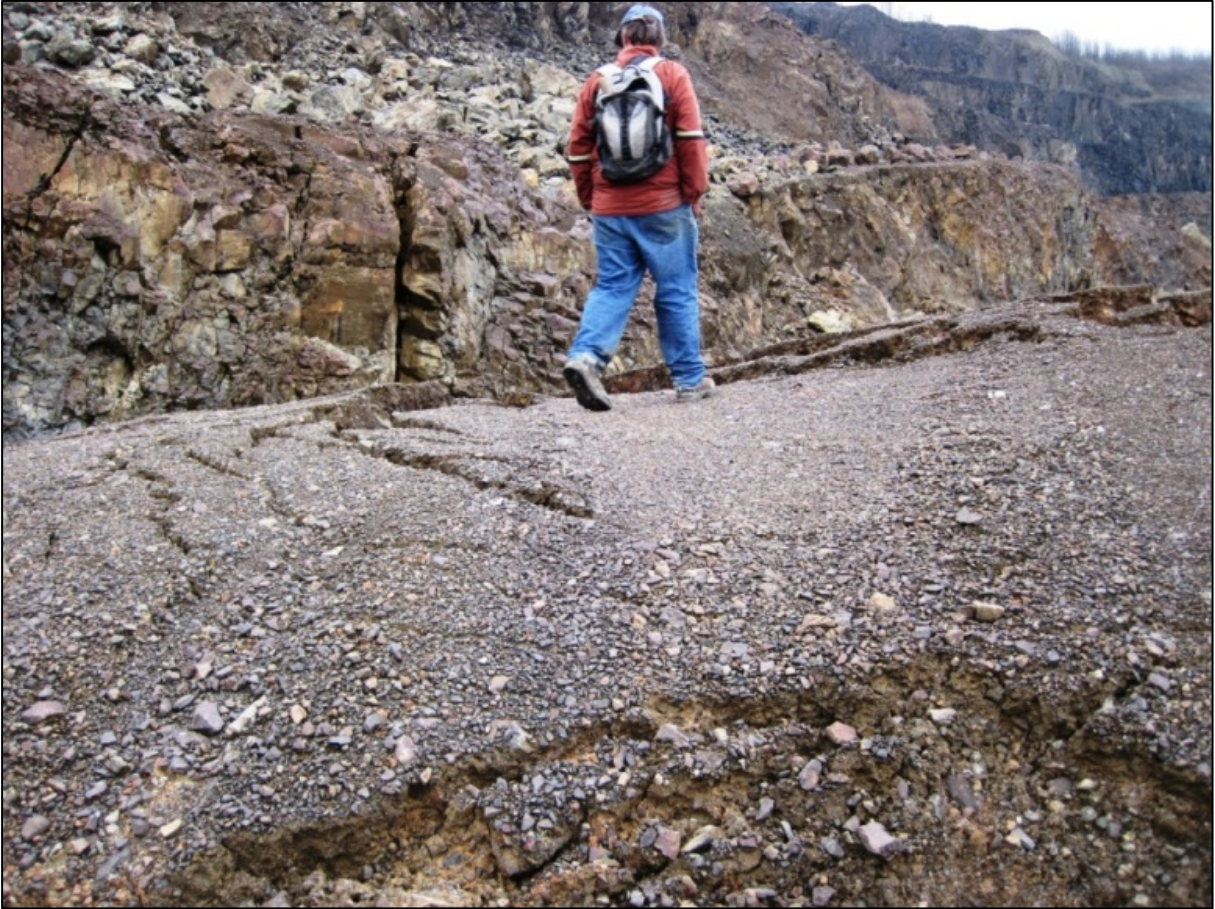
Figure 5. Bedrock landslide on the east wall. This pressure mound is about 4 ft high on the north portion of the slide.
