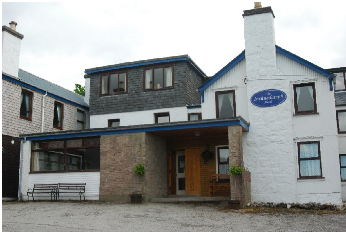
Figure 8. The historic Inchnadamph Hotel in Assynt.
