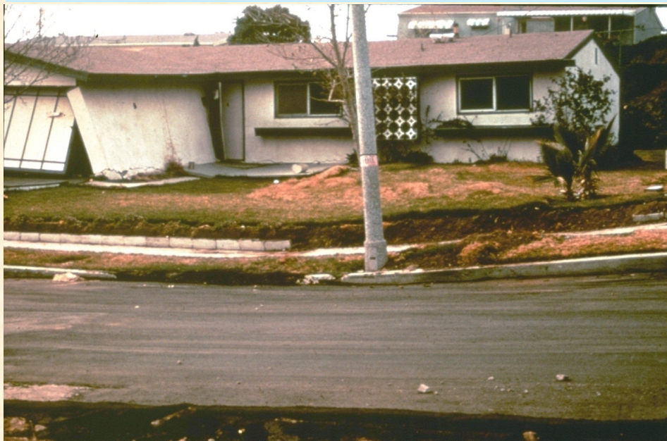
A single family residence damaged by fault rupture. The location of the fault is evident in the sloping sidewalk and crumpled lawn. Photo credit: Earl Hart, CGS.
